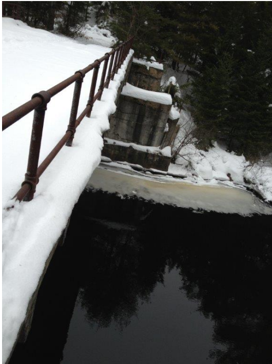
Goodman Bridge/ Concrete Bridge
